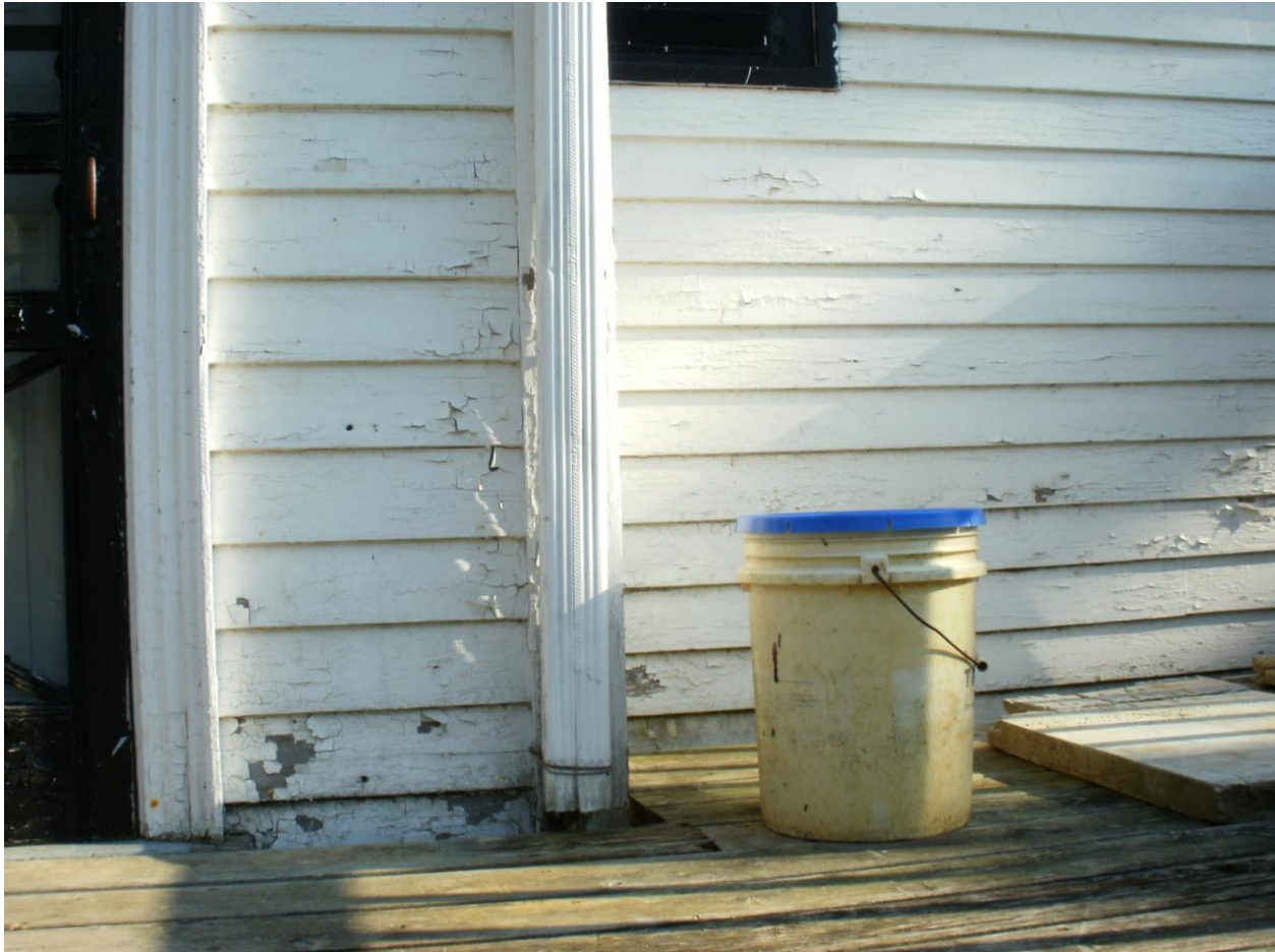
Figure 1: The gutter on the north wall, possibly causing the leak in the cellar.
