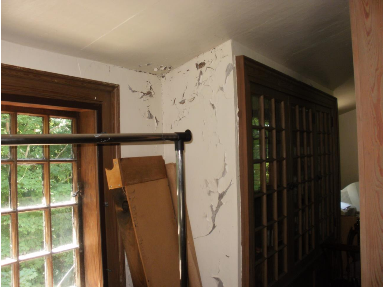
Figure 2: Water damage to the south wall, possibly from a leak around the chimney. Water damage is also evident inside the wall of the adjacent built-in cabinet.
