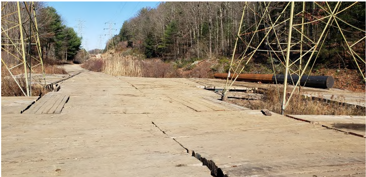
Photo 2: Work pad at Structure 10103 (on right) on November 15, 2019 after installation of caisson (looking north).
