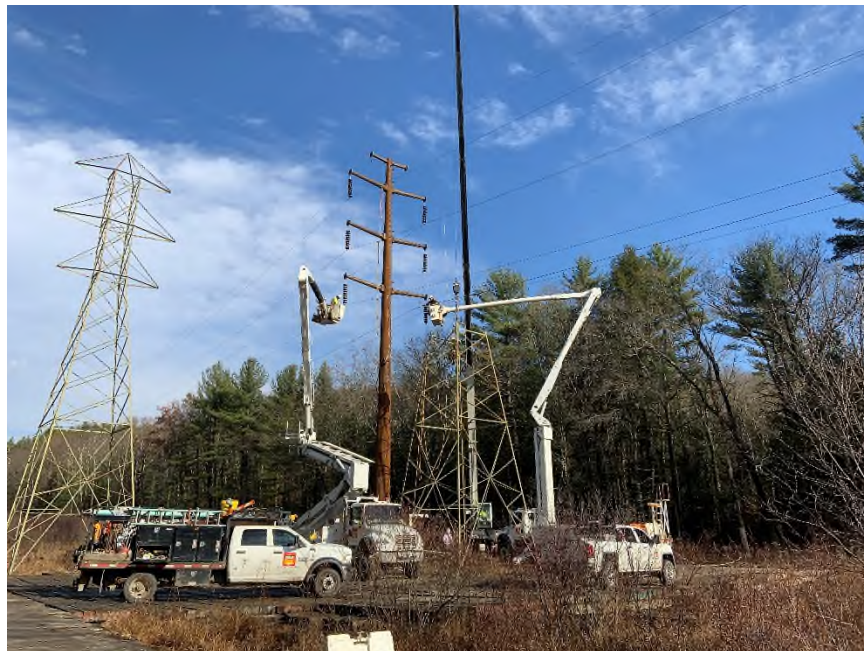
Photo 4: Installation of new Structure 10104 on November 25, 2019.
