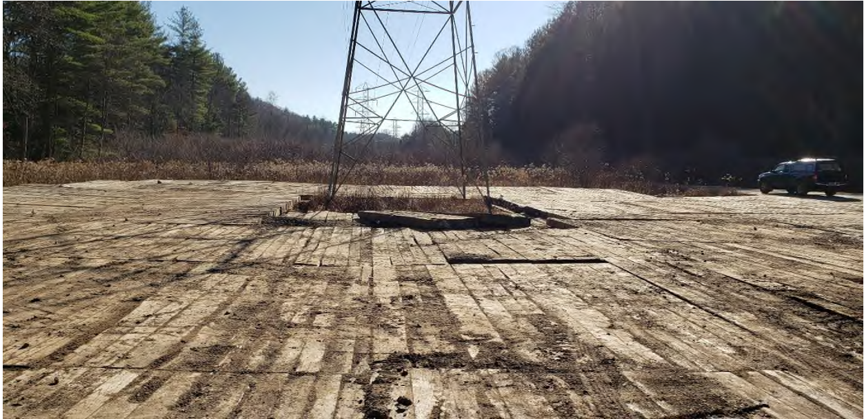
Photo 1: Work pad at Structure 10104 on November 15, 2019 after installation of caisson (looking south).
