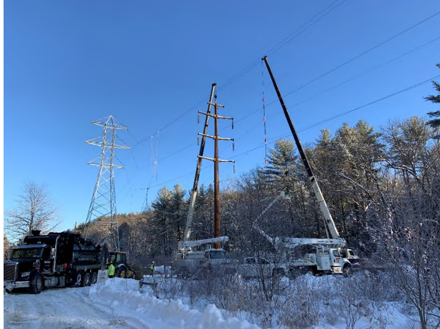
Photo 6: Lifting newly installed Structure 10104 on December 7, 2019.
