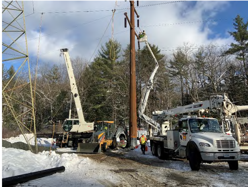
Photo 7: Reinstalling the lines to the insulators on Structure 10104.
