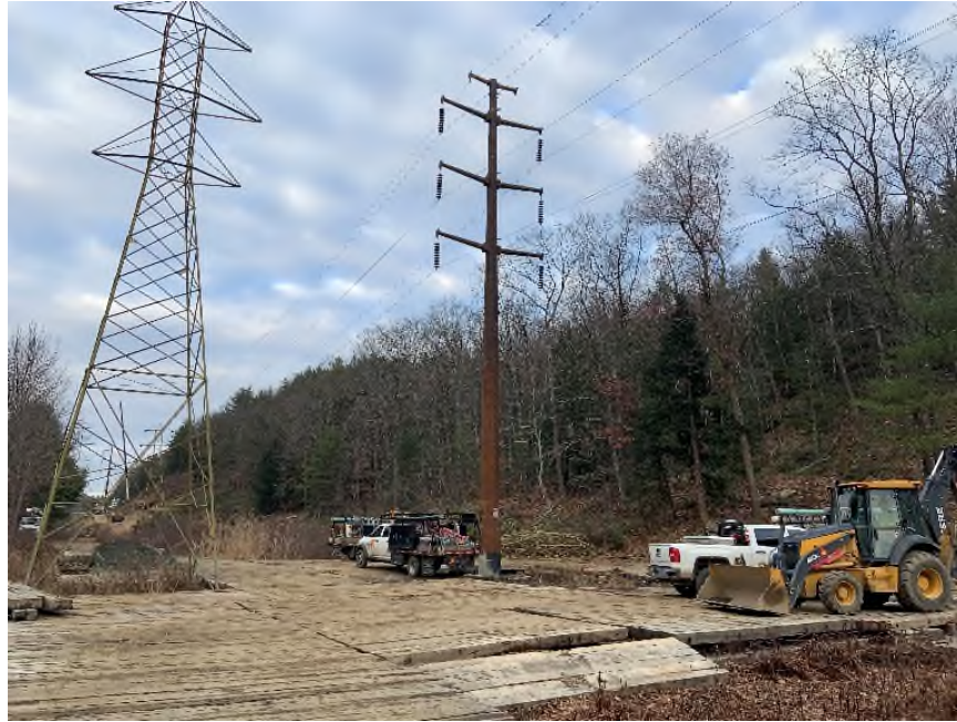
Photo 3: Completed Structure 10103 installation on November 25, 2019.
