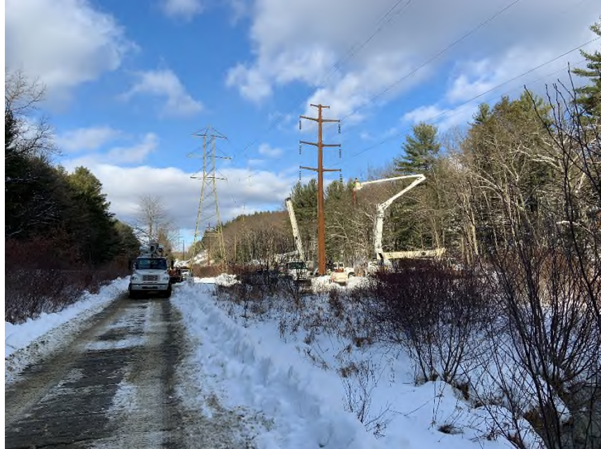
Photo 8: Completing the reinstallation of Structure 10104 on December 7, 2019.
