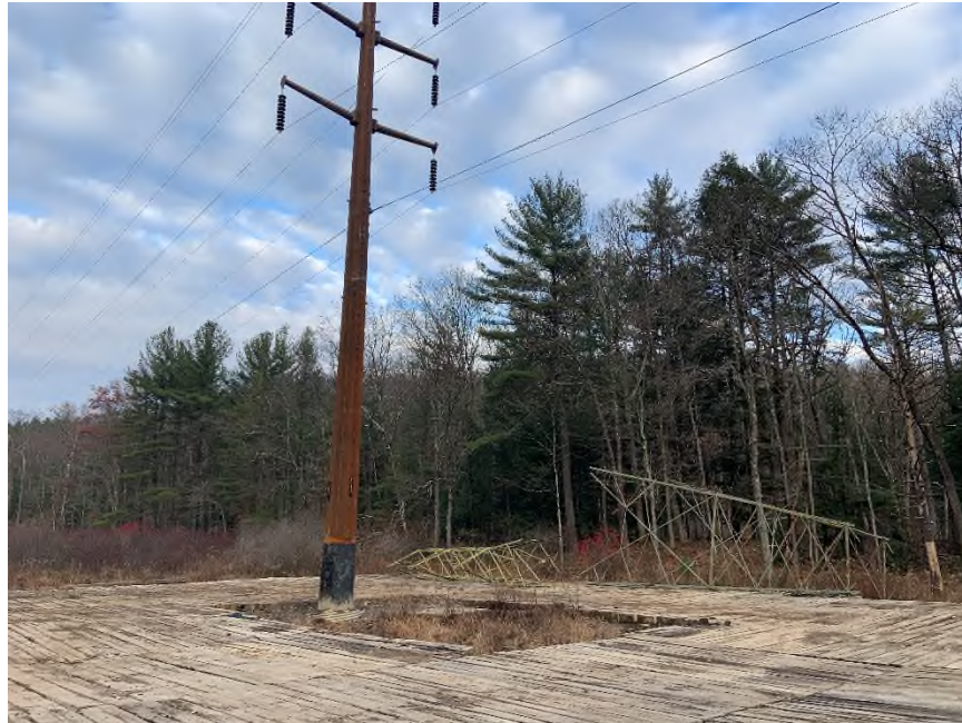
Photo 5: Completed installation of Structure 10104 on November 25, 2019. Old lattice structure on the work pad.
