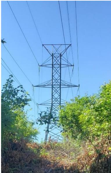
Typical metal lattice frame structure
