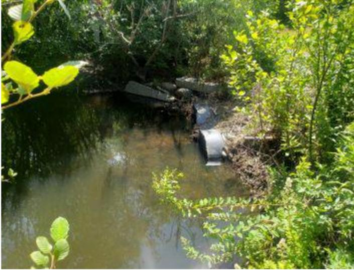
View looking west at culverts. Water is below flood level, but accumulated debris indicates limited flow through this area.
