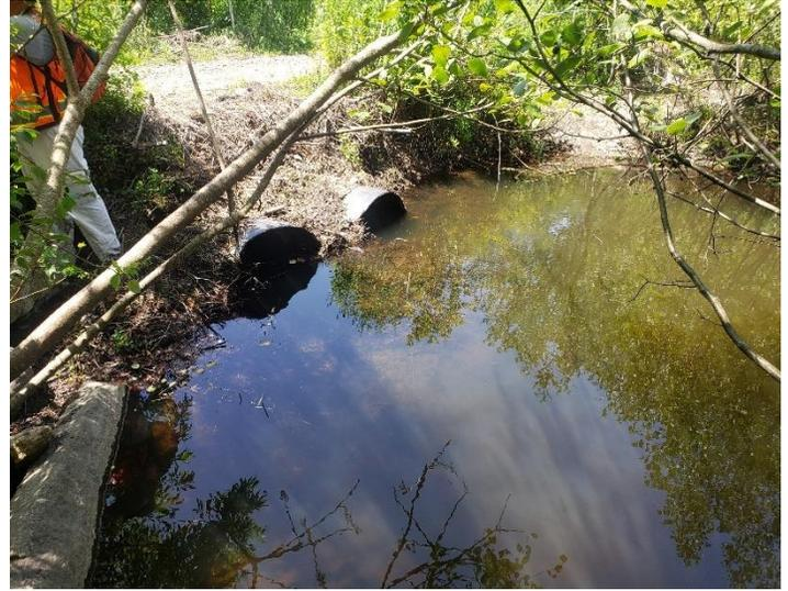
View looking northeast at culverts. Water is below flood level; however, scour path is visible to the right of the culverts which results in access road flooding.
