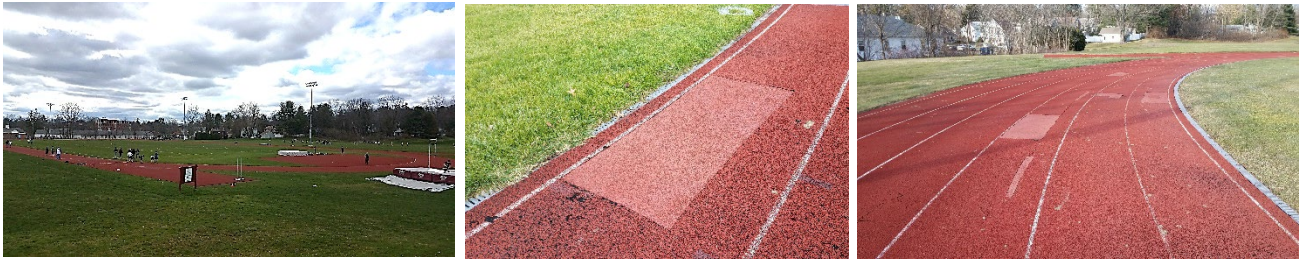
Overall image of Track and Multi-Use Field 1 (left photo), the poor surface condition (middle photo,) and the consistent cracking and damaged areas of the track (right photo) have resulted in the track being unusable for league and tournament meets. Note the lack of ADA accessibility at the site as shown in the panoramic photo on the previous page.
